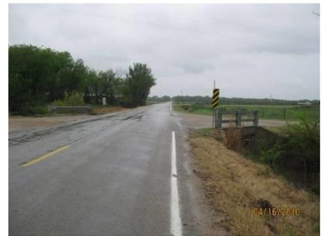
Many of the culverts on intersecting roads and entrances represent essentially a blunt object when impacted by a vehicle. These “parallel” culverts can be mitigated by either relocation to a location where it is less likely to be impacted or installation of a traversable grate. For this category we propose allowing use of HRRR funding for a county to address culvert issues, either on a corridor-wide or site-specific basis, without being required to provide site-specific crash data.
