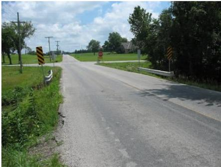
are tree and barrier removal, lengthening culverts to allow for drivers to recover can help reduce the sixth most common reason for ROR fatalities. Another alternative would be to install traversable grates over the end of the culvert.
