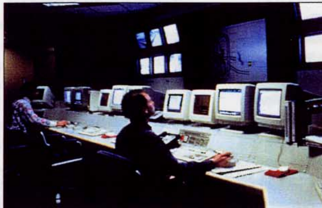
Traffic Operations Center
