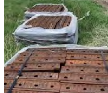
Materials for construction wait to be installed.
