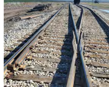
Completed slider track.
