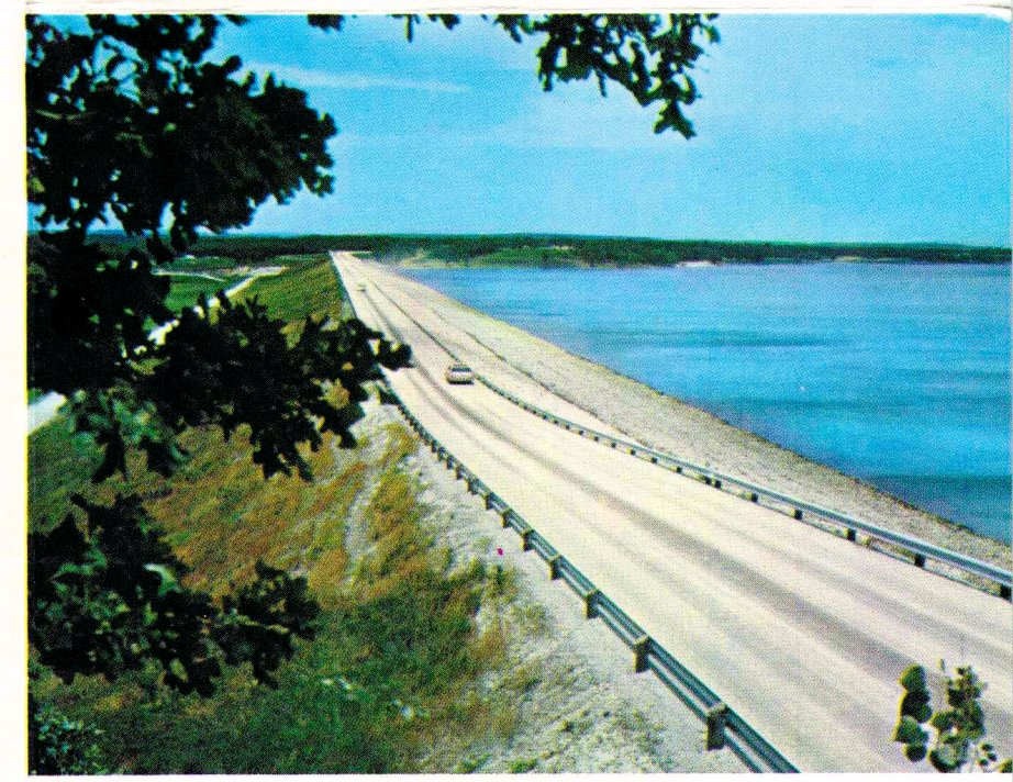
Access Road—Toronto Reservoir
