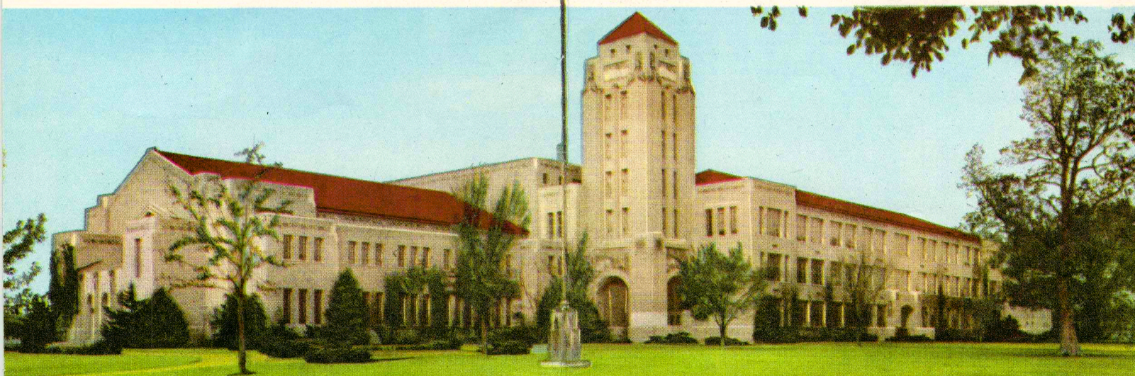
Shrine for Education; Prize-Winning Architec- ture in Wichita High School North, near US-81, 54; K-15, 96
