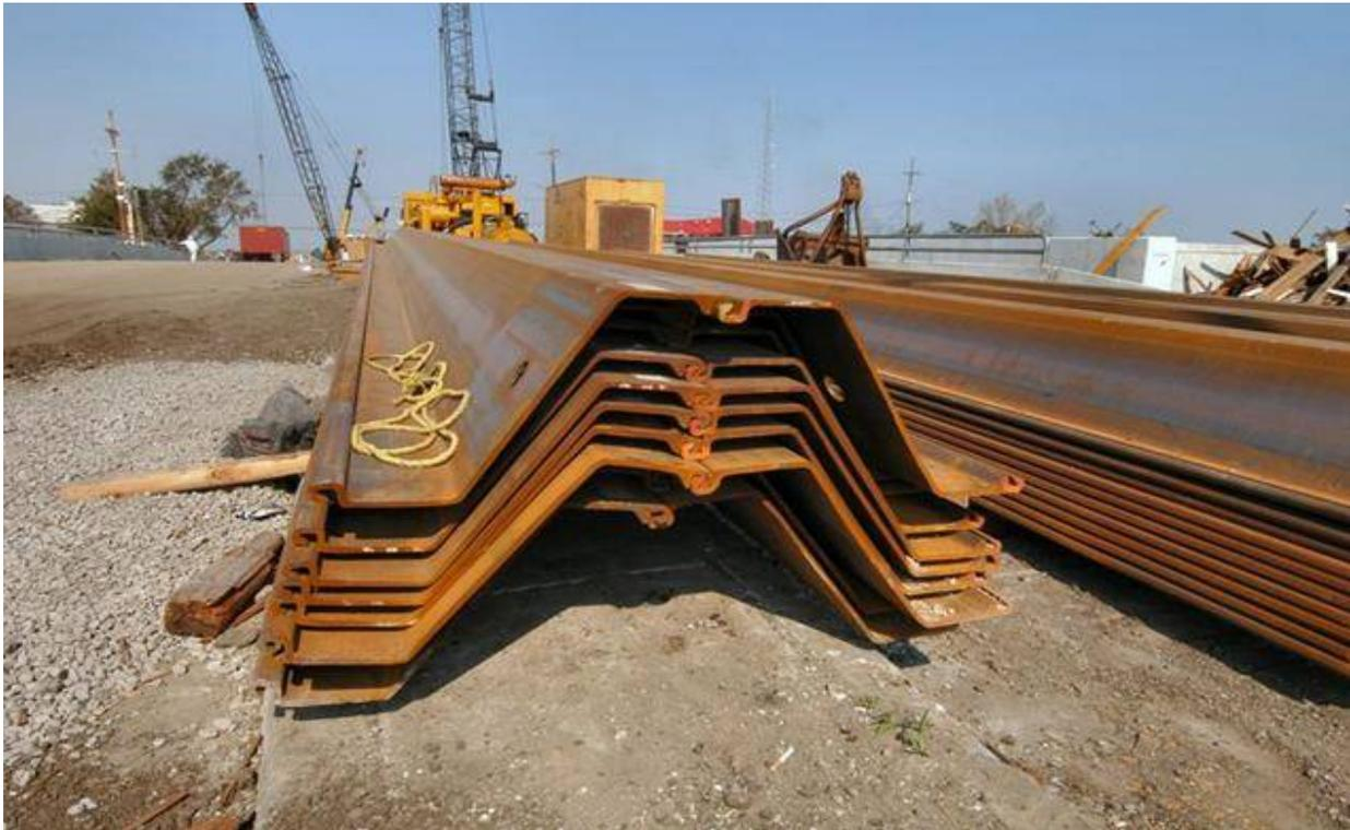
**Figure 4: Pre-coupled Z-shape Sheet Pile**
