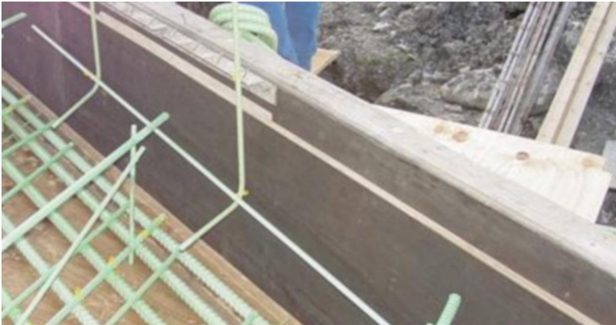
**Figure 20:  $\frac{3}{4}$ " Triangular Chamfer Strip**
