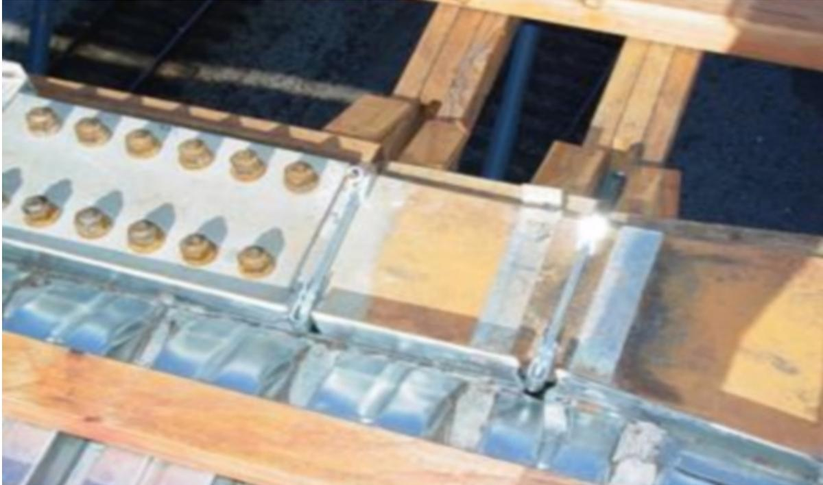
**Figure 13: Steel SIP Forms and Welded Support Hangers**
