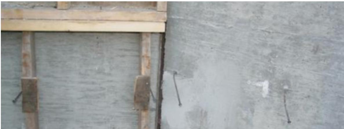
**Figure 10: Remaining Break Off Ties**
