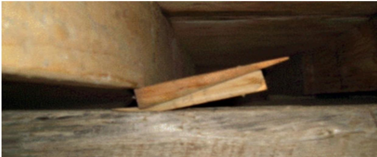
**Figure 20: Incorrect Shim Placement**
