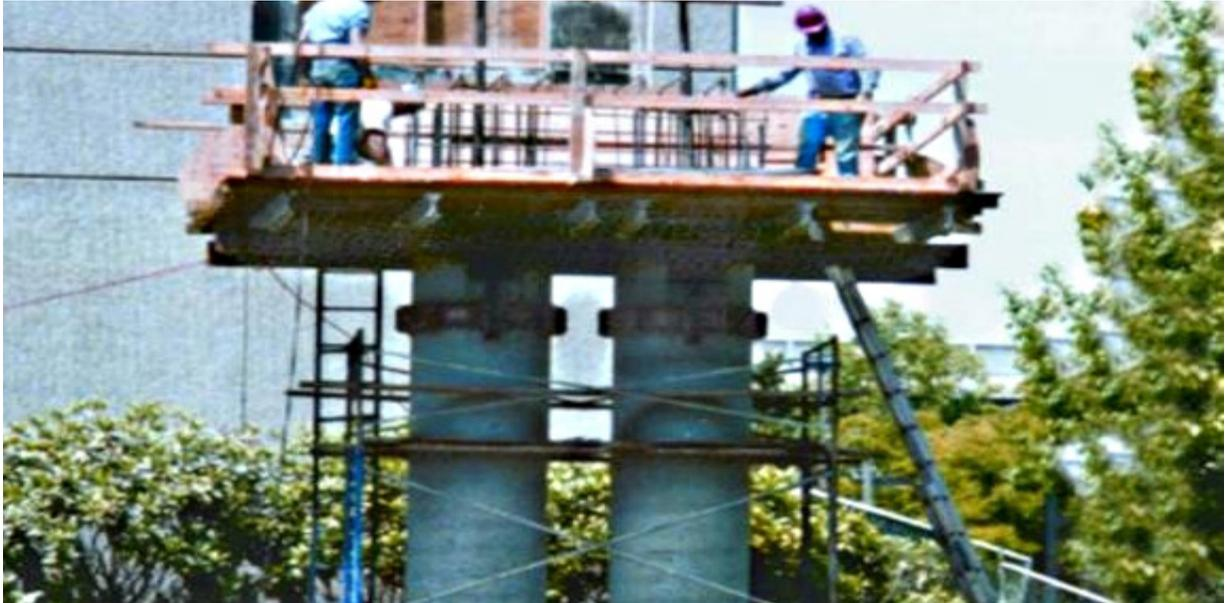
**Figure 17: Friction Collars Attached to Columns**
