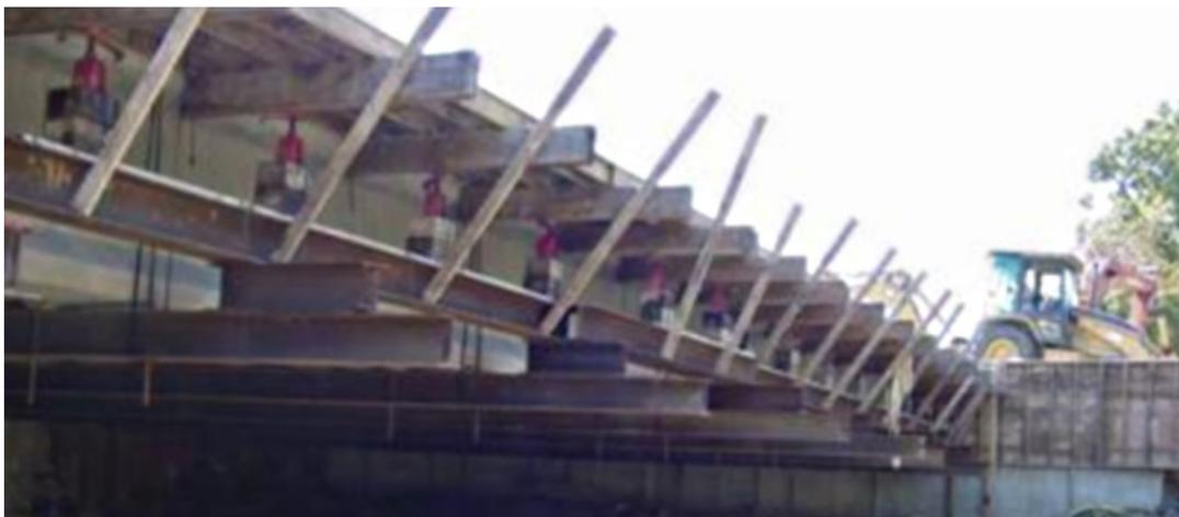
**Figure 8: Needle Beam Overhang Falsework**
