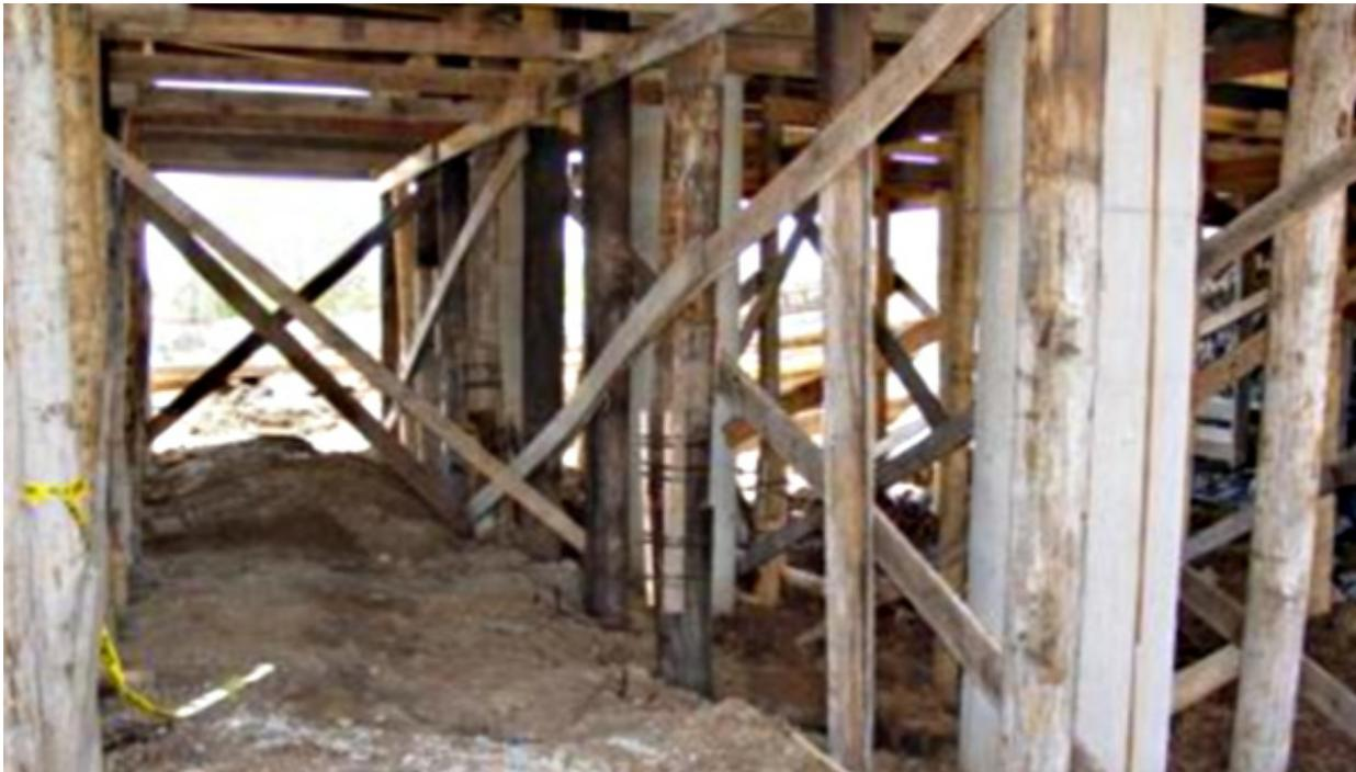
**Figure 18: Falsework Column Splice (Center)**
