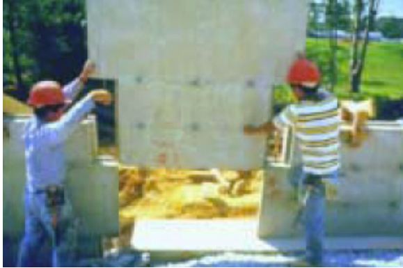
Figure 5, Placing Panels
