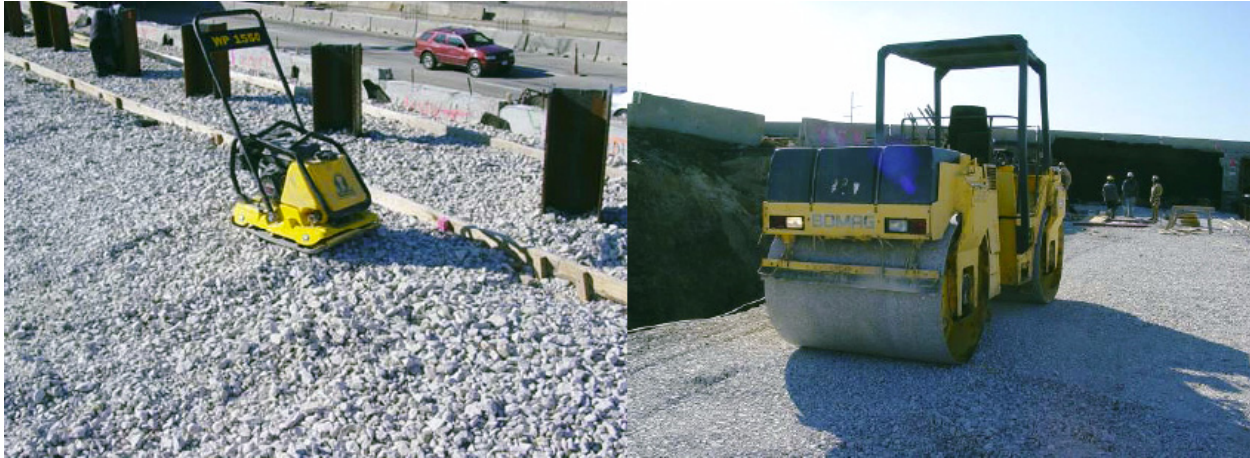
Figure 20, Compaction Equipment
