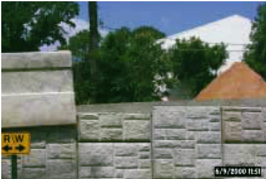
Figure 15, Leveling Course for Coping/Barrier
