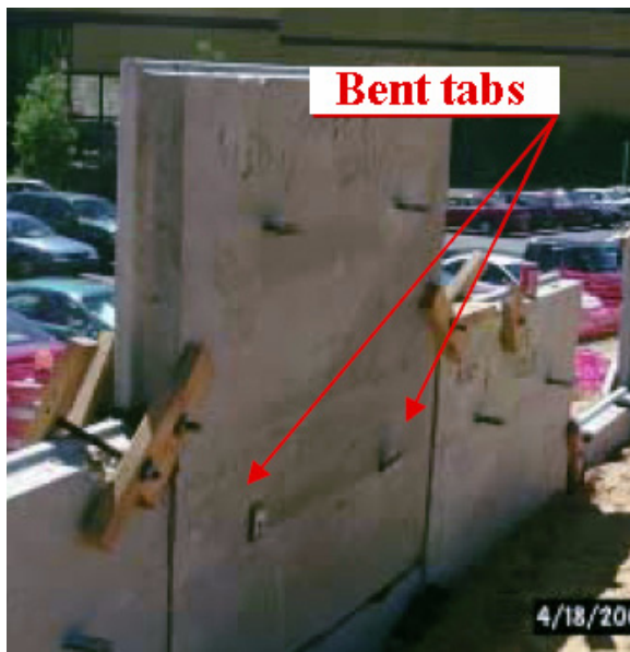
Figure 10, Damaged Tabs
