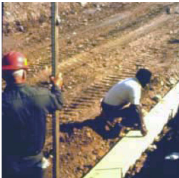
Figure 3,Leveling Pad
