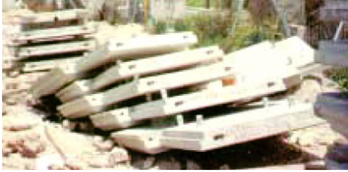
Figure 9, Improper Panel Storage
