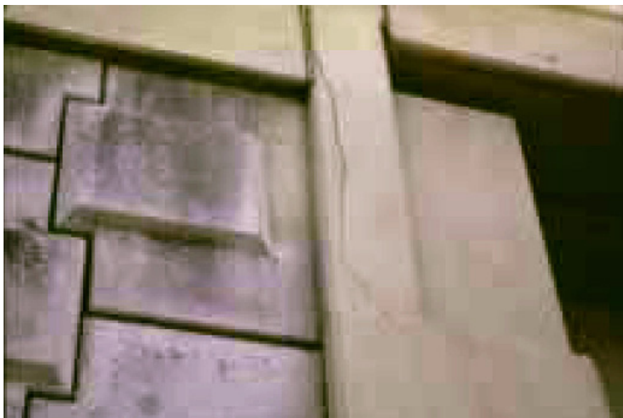
Figure 19, Tension Break in Cheek Wall
