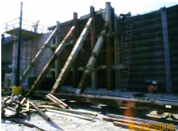
Figure 29, Temporary and Permanent Wall Facings
