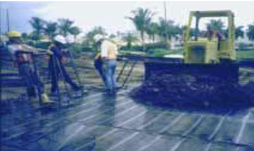
Figure 37, Tensioning Polymer Reinforcement
