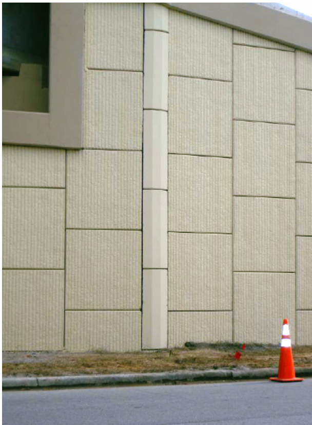
Figure 6, Slip Joint
