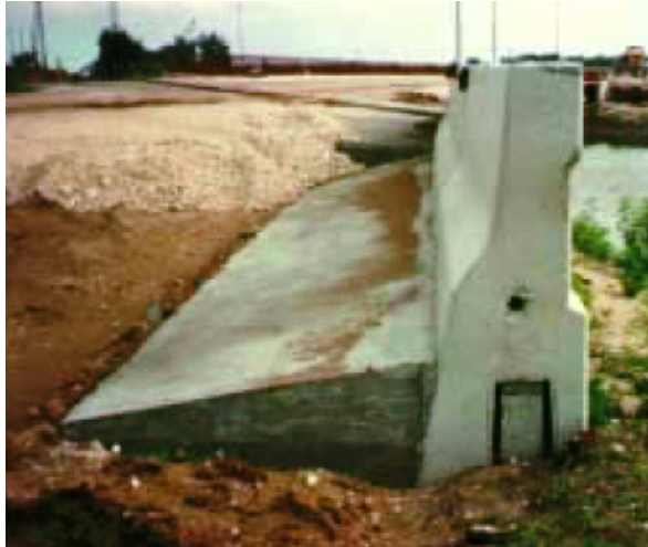
Figure 16, Barrier with Slab
