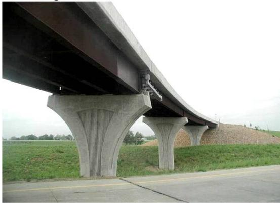
Steel Welded Girder Haunched-SWGH
