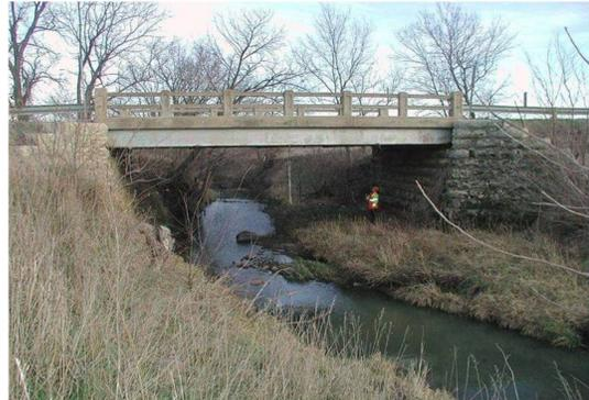
Weathering Steel Welded Plate Girder Continuous-WWGC
