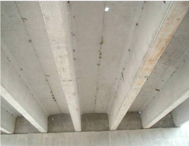
Prestressed Concrete Beam Continuous-PBMC
