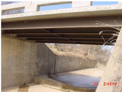
Steel Riveted Girder Continuous - SRGC
