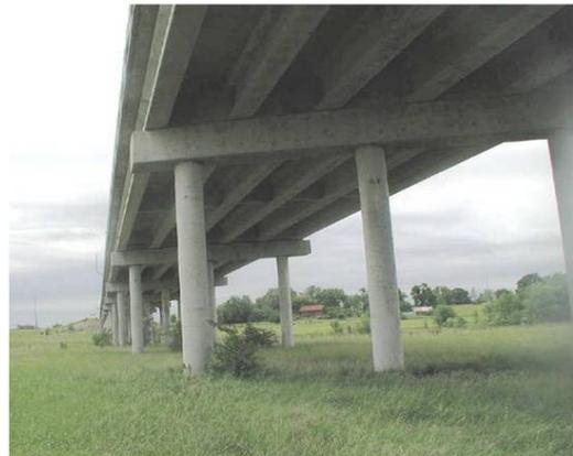
Column Bent with Web Wall on Drilled Shafts
