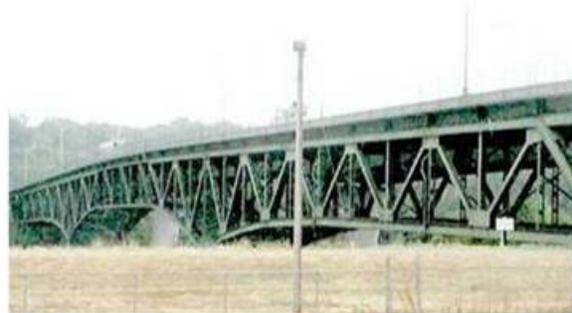
**Steel Deck Truss Continuous - SDTC**
