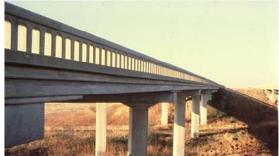
**Reinforced Concrete Open Spandrel Arch Fixed - ROAF**
