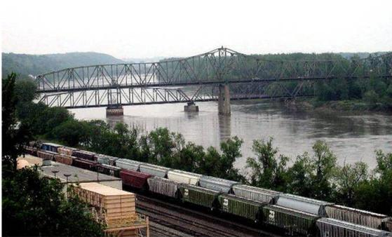
**Steel Low Truss Simple - SLTS**
