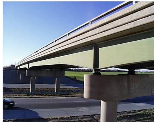
Steel Welded Girder Simple - SWGS
