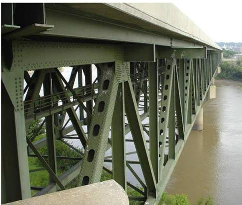
**Steel Low Truss Continuous – SLTC**
